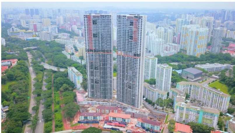
Figure 2.21. Avenue South Residences (BCA Singapore, 2022a)
