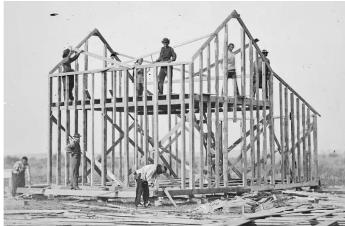
Figure 2.3. Balloon frame house, Omaha Reservation, Nebraska, 1877 (Huets, 2013)
