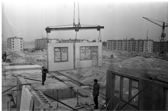
Figure 2.9. Prefabricated panel construction in 1961 and 1964 (Malaia, 2020)
